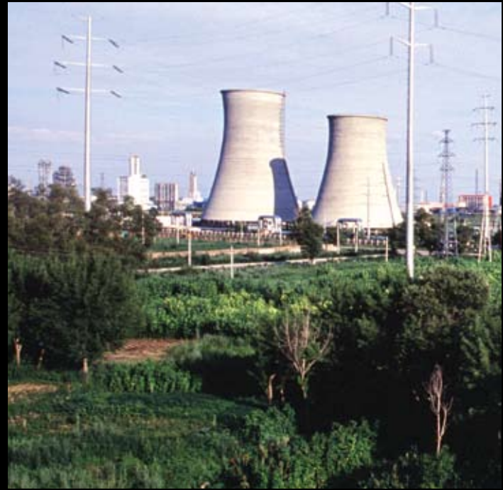
The Daqing Hongwei thermal power plant in Daqing, Heilongjiang
